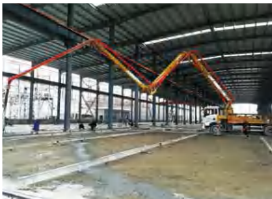
30米泵车厂房内施工 (30米泵车厂房小试牛刀) HB30K boom pump is trying its hand at the workshop.
