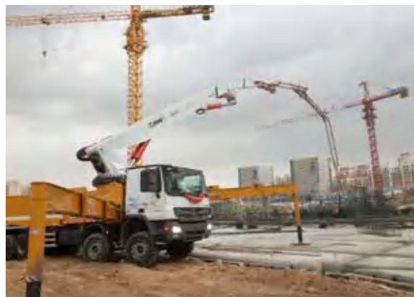
HB62V 泵车江苏展雄姿 HB62V boom pump is exhibiting its manhood in Jiangsu
